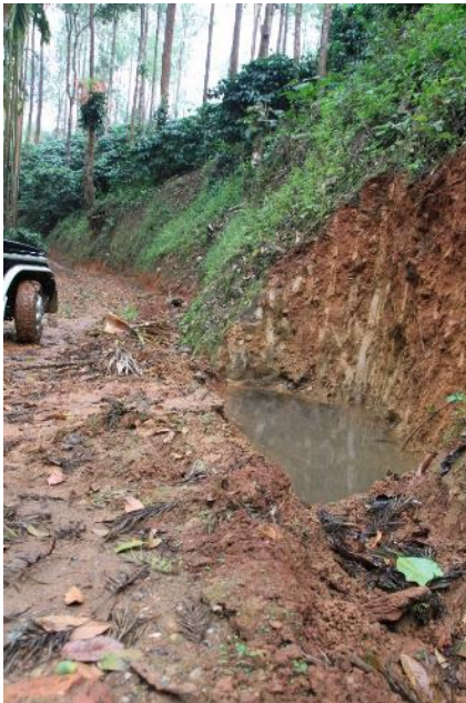
Figure 5. Soil and water collecting pits dug along the estate roads
